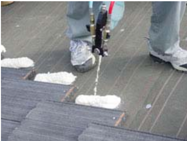
Figure 5: SPF Adhesive patty application.
