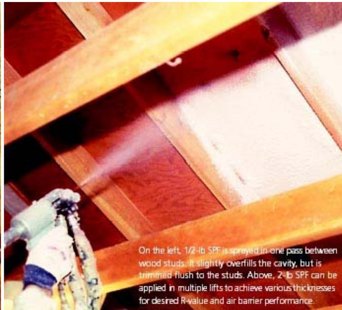
On the left, 1/2-lb SPF is sprayed in one pass between wood studs. It slightly overfills the cavity, but is trimmed flush to the studs. Above, 2-lb SPF can be applied in multiple lifts to achieve various thicknesses for desired R-value and air barrier performance.
