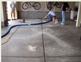
Raising-Leveling-Void Filling
