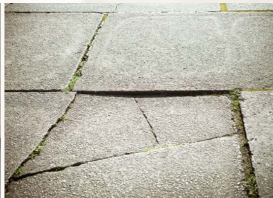
Concrete Lifting
